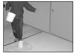
*Tip:* To achieve a uniform chip coverage, toss the chips upward over the freshly coated area.
