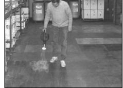
garden sprinkling can as uniformly as possible. Allow Etcher to work for 5 minutes. Scrub with low speed floor machine equipped with a grit brush. Pick up solution with a wet/dry vac or squeegee solution into floor drain. An automatic scrubber may also be used.
